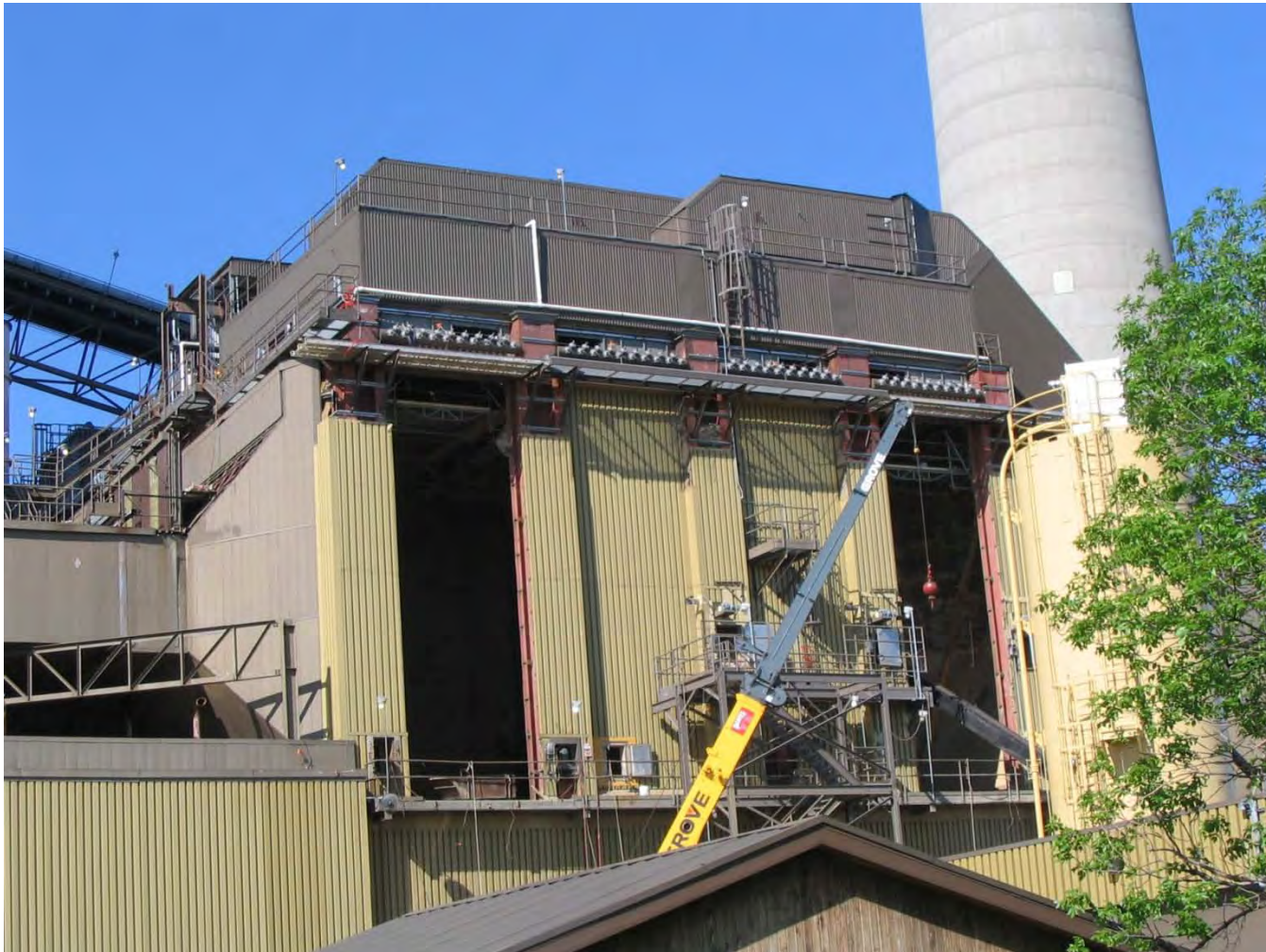
ESP Side Cut-outs for ESP internals Demolition
