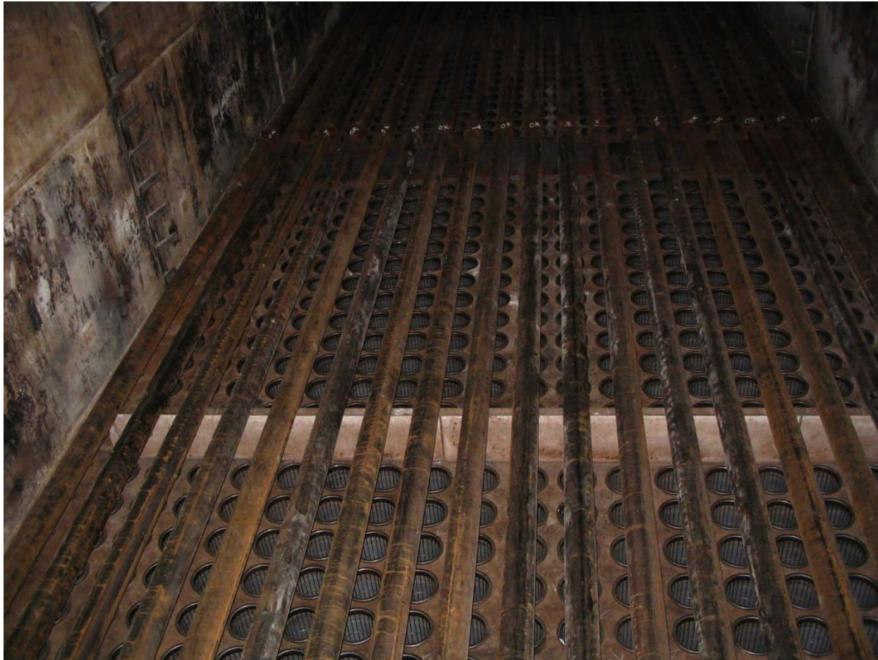
Big Stone Compartment Tubesheet
