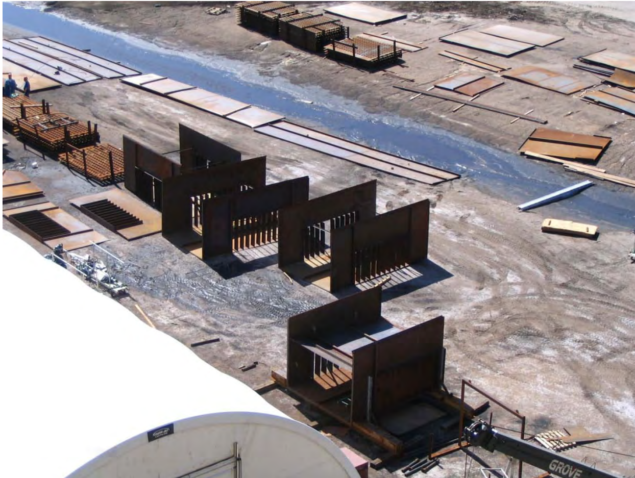
Pre-Assembly of Inlet Plenum Sections
