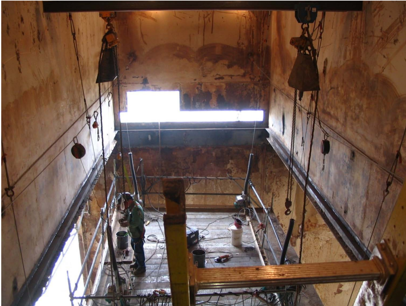
Compartment Tubesheet Shelf Installation
